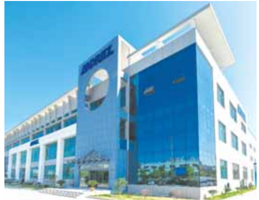
The new ANDRITZ Nonwoven facility in Wuxi, China.
