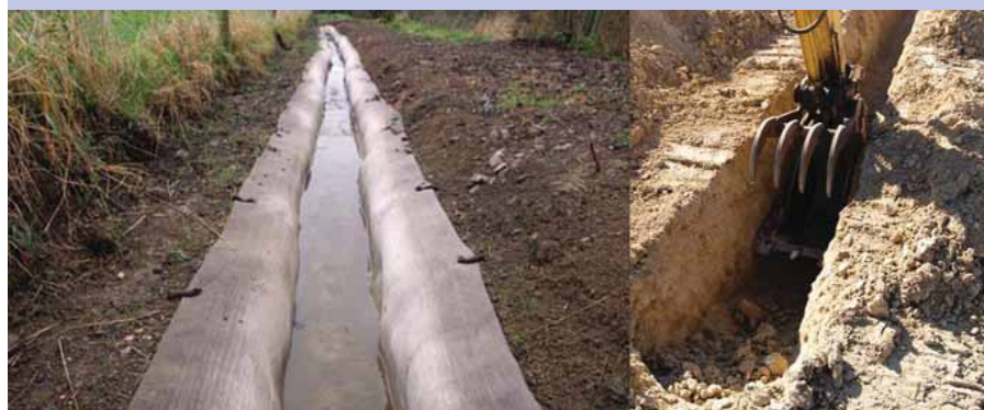
Concrete Cloth: Can be rapidly unrolled to form ditch or tank lining.
