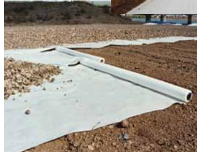
Geotextiles can extend the life of the road and decrease its immediate and life time cost.
