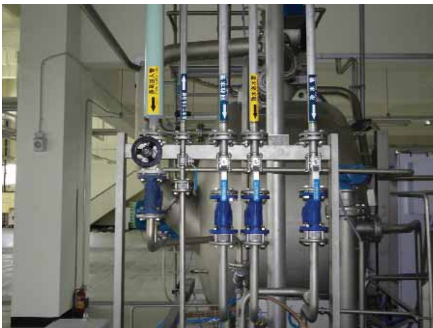
The stainless steel pipe work system offers easy connection to the mains utilities with reduced installation costs.
